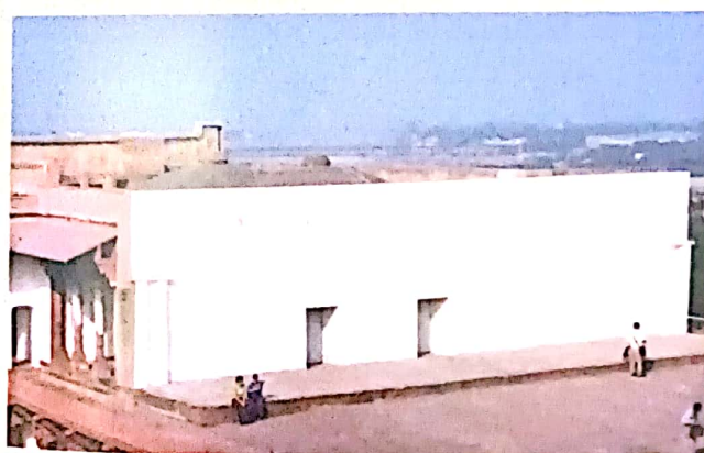
Exterior view of Shahi Hammam
