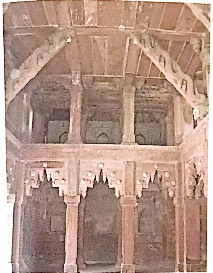
Jahangiri Mahal interior view
